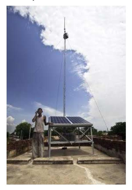
WorldGSM is a communications-based station in India owned by Vihaan Networks Limited (VNL), which uses some solar panels for its entire operation without connecting to the grid. The solar-powered cell phone towers will use Boston Power batteries to power the tower, which could set its use up to 3 days without
